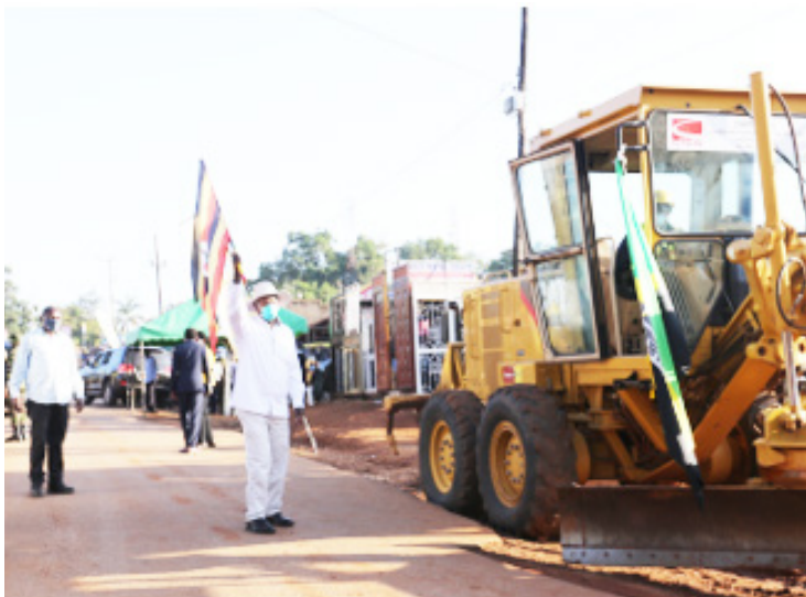
Commissioning the road works
